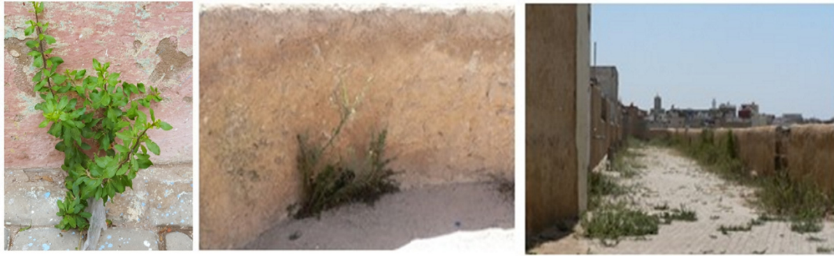
Fig. 7. Proliferation of vegetation at the base of the walkways walls of the Portuguese city.
