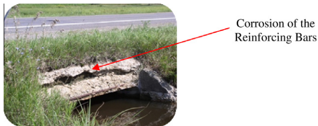
Figure 7 Condition of culvert structure 31000131B05.
