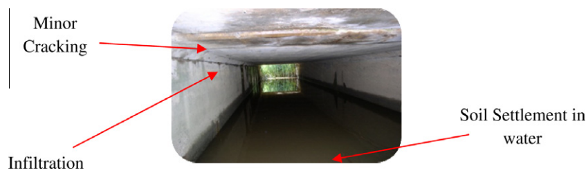
Figure 5 Condition of culvert 31000131B04.
