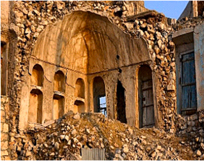
Fig. 5. Cover system of Siirt Houses (Author – 2020).
